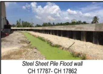
Steel Sheet Pile Flood wall
