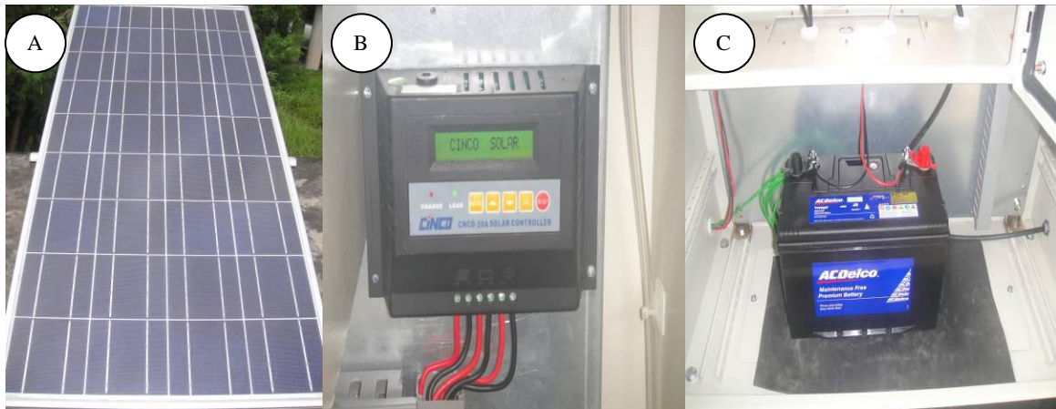
Gambar 2: A) Panel Solar, B) Solar Charger Regulator, C) Bateri 12 watt 100A
