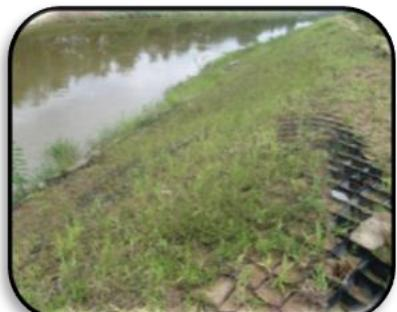
Geoweb Earth-filled Lining
