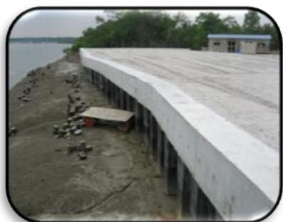
Steel Sheet Pile Wall
