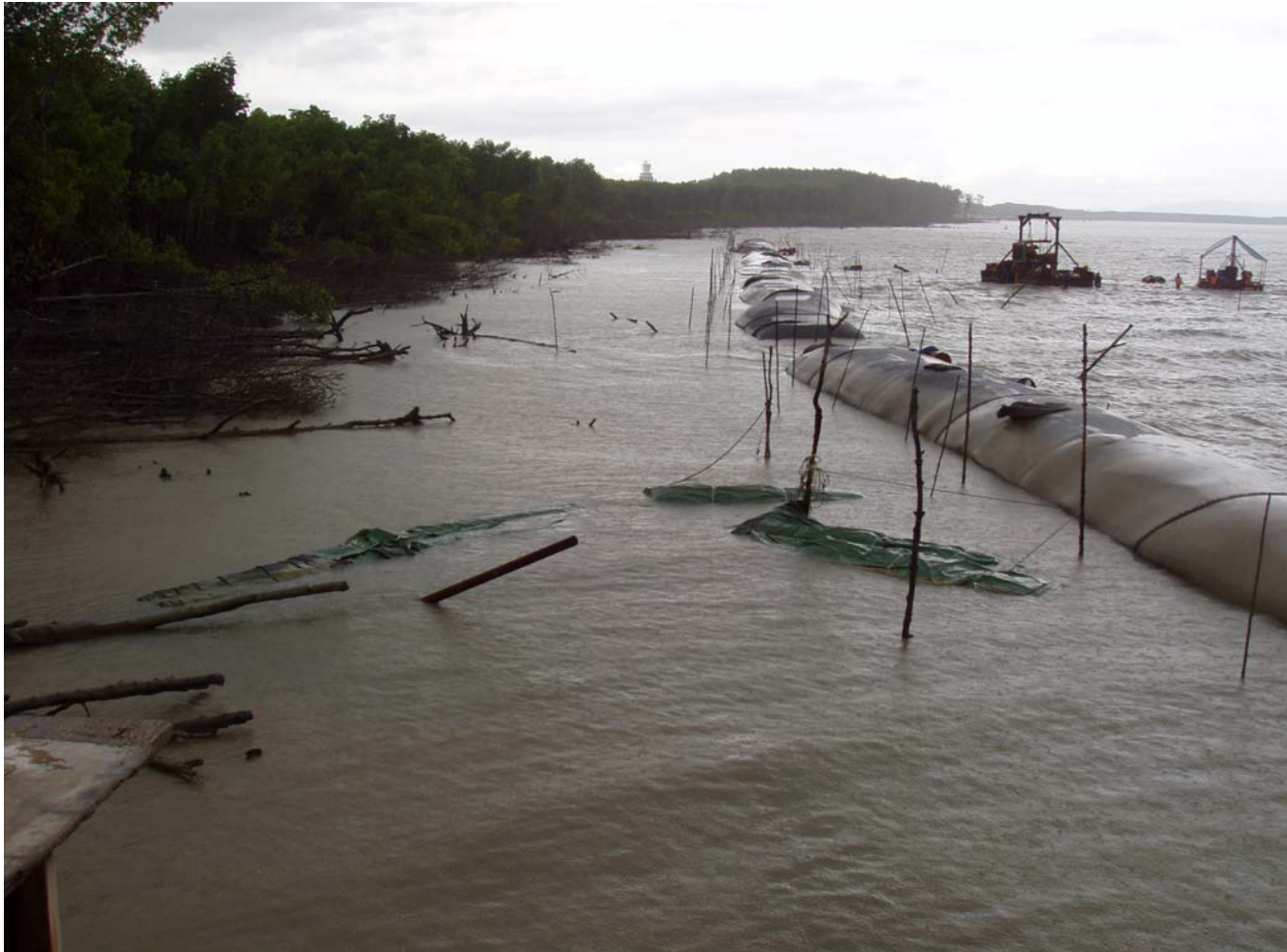
Figure 5: Sand-filled Geotextile tubes placed in front of eroding mangrove shoreline
