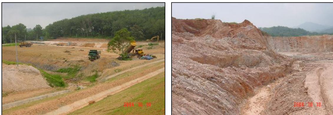
Figure 1.1: Large-scale earth works without erosion control BMPs
