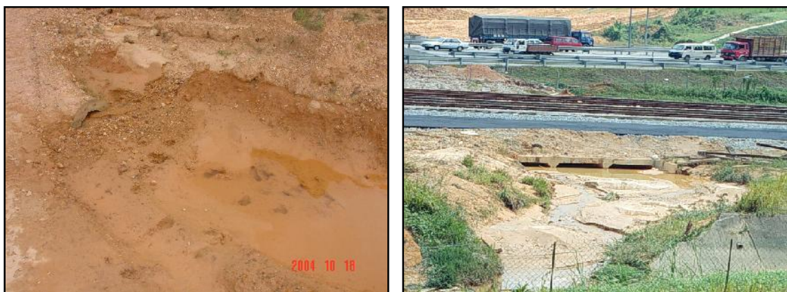
Figure 1.2: Consequent severe sedimentation of drains and culverts downstream
