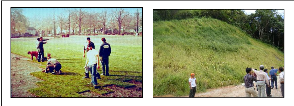
Figure 5.1: Examples of seeding and turfing
