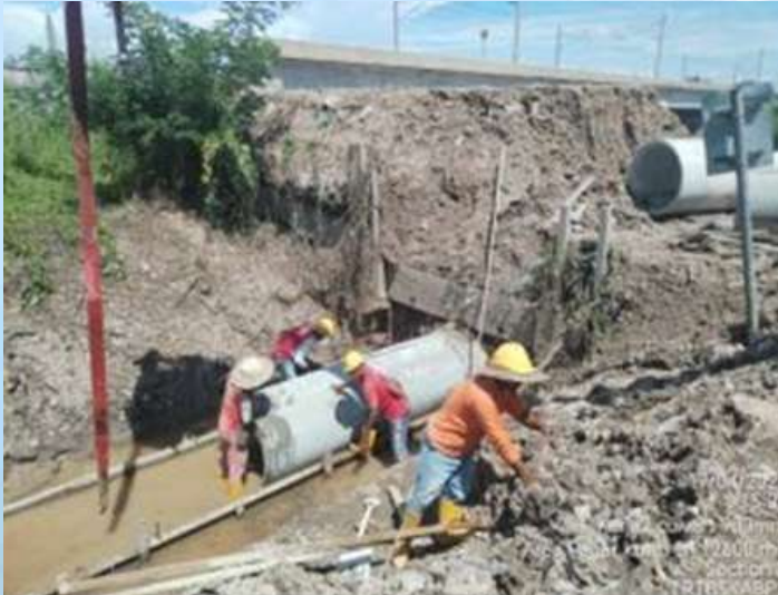
Kerja-Kerja Drainage Outlet Structure CH12600 RHS
