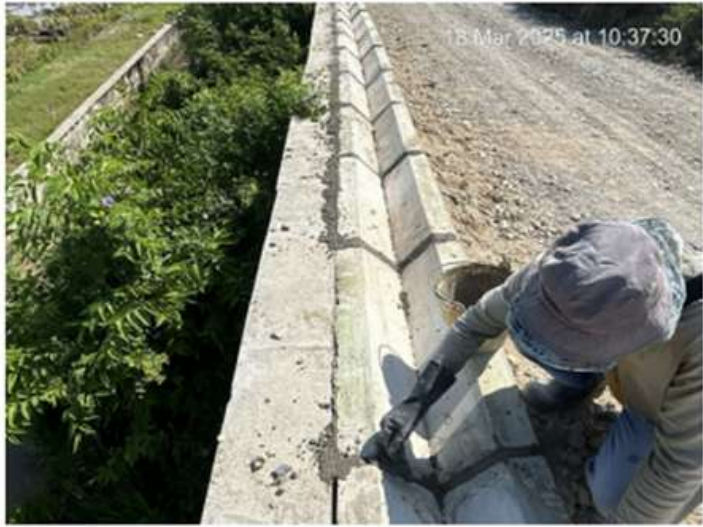
Filling Works LTB Crossing CH12250
