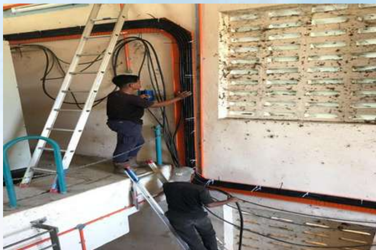
Dismantle Existing Motor Power Supply Cable
