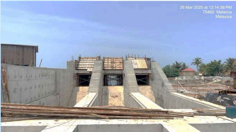
Pump Station Parit Kiri: Main Structure Pump Support Beam
