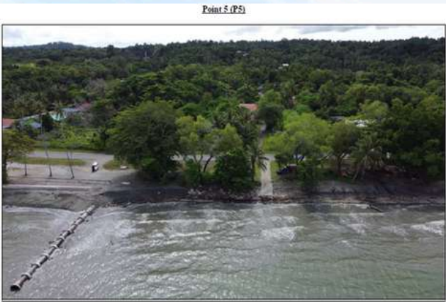
Gambar 6 : Beach Nourishment, Seawall dan Marine Outfall No.3
