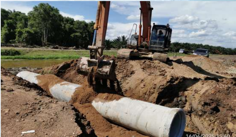
Outlet Structure: Sungai Ayer Molek
