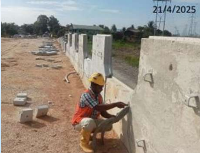
Kerja-Kerja Ramp JKR Bridge CH9600 RHS
