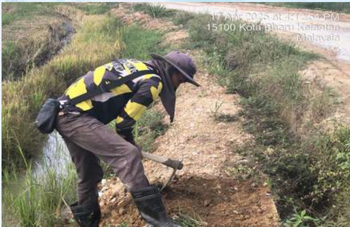
KADA Irrigation (Site Seribong) Kerja-Kerja Pembersihan Pre-Cast U Drain Irrigation
