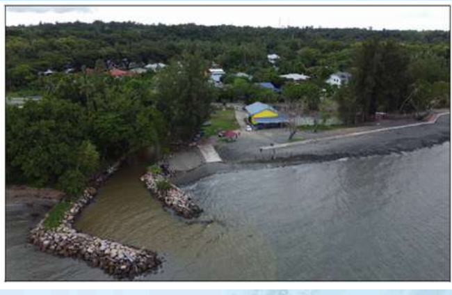
Gambar 2 : Ramp, Rock Revetment, Seawall dan Beach Nourishment
