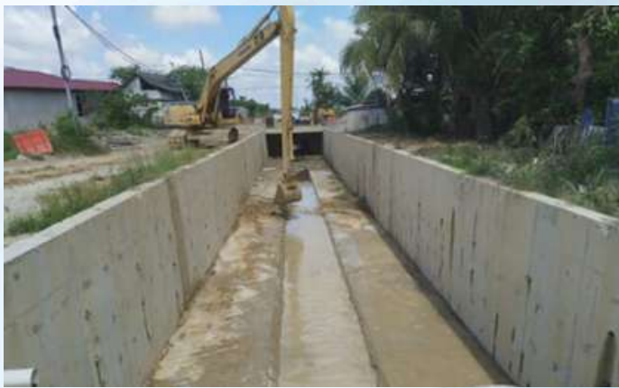
Seribong Main Drain – Kerja-Kerja Mencuci Concrete Channel CH1400 – CH2230
