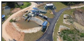
Aerial View Rumah Pam Bagan Samak
