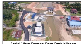
Aerial View Rumah Pam Parit Nibong
