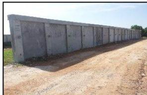
Well guard Flood Wall
