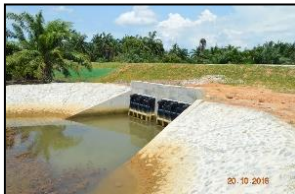
Control Outlet Structure (Twin) CH 10650
