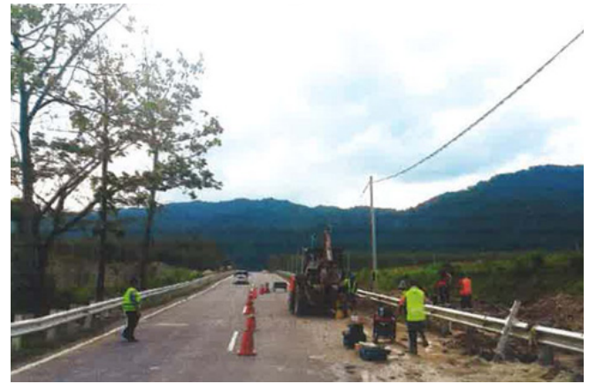
Sambungan Kerja-kerja Lay Cable Joint Cable
