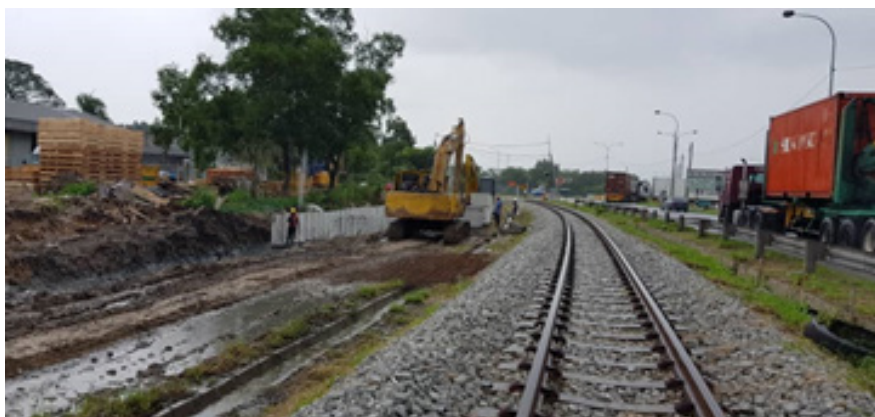
SUNGAI DUA BESAR, NORTHPORT - Interlocking Pavement & Railing
