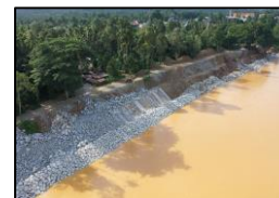
Kg. Temangan River Protection Works
