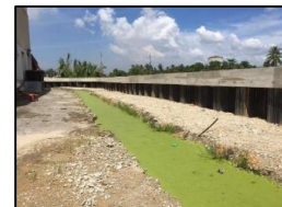
Steel Sheet Pile Flood Wall CH17787 – CH17862
