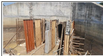
Inlet Structure CH10200
