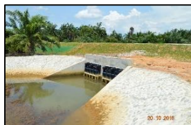
Control Outlet Structure (Twin) CH10650
