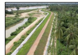
Kg. Gerong Flood Levee
