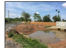
Drainage Outlet Structure CH19150
