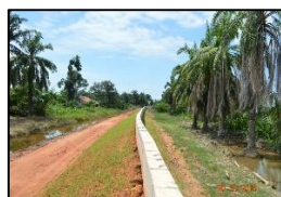
Flood Wall CH700 – CH8300
