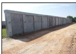
Well Guard Flood Wall
