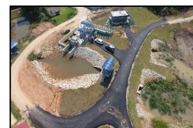
Aerial View Rumah Pam Bagan Samak
