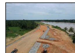
Kg. Gerong Flood Levee
