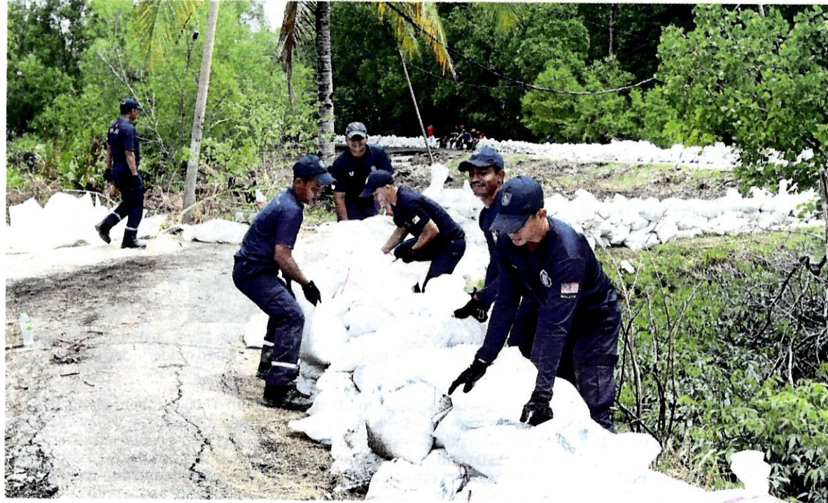
The Special Malaysian Disaster Rescue Team (SMART) stacking sandbags at Kampung Tok Muda, Kapar.
