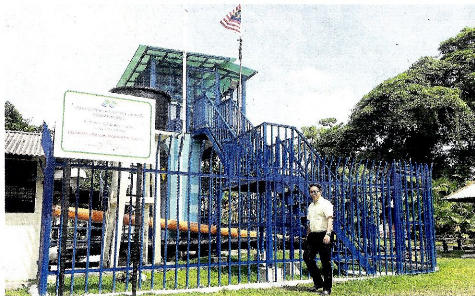
Leong says sluice gate No. 38 at Jalan Tepi Sungai, that helps to avert floods, is on alert mode for the high-tide phenomenon
