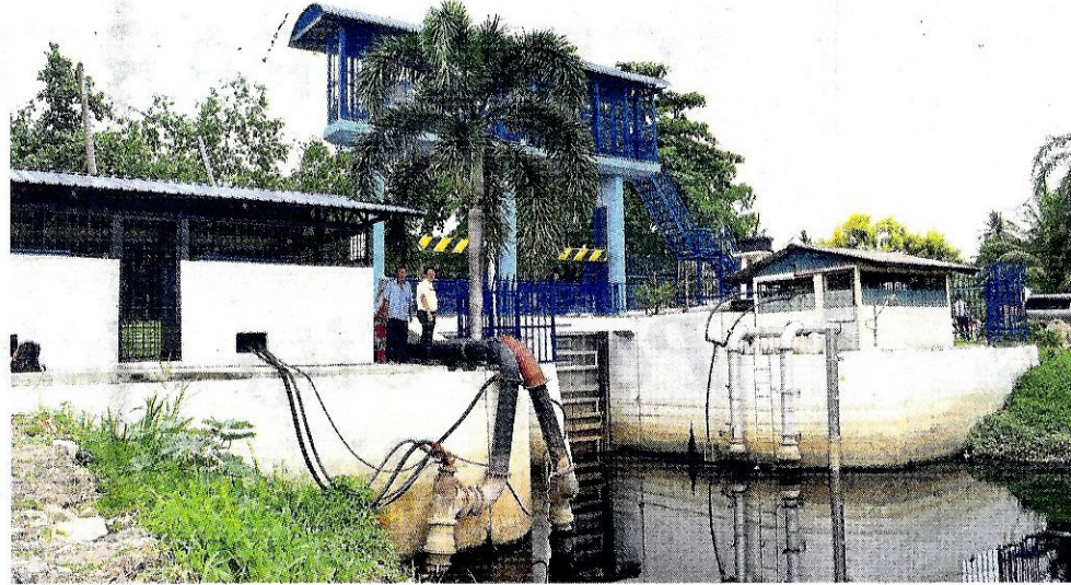
The existing Teluk Gadong Besar Sluice Gate 44 that helps control flash floods for 10 neighbourhoods in Klang. A new sluice gate is expected to be built next to it.
