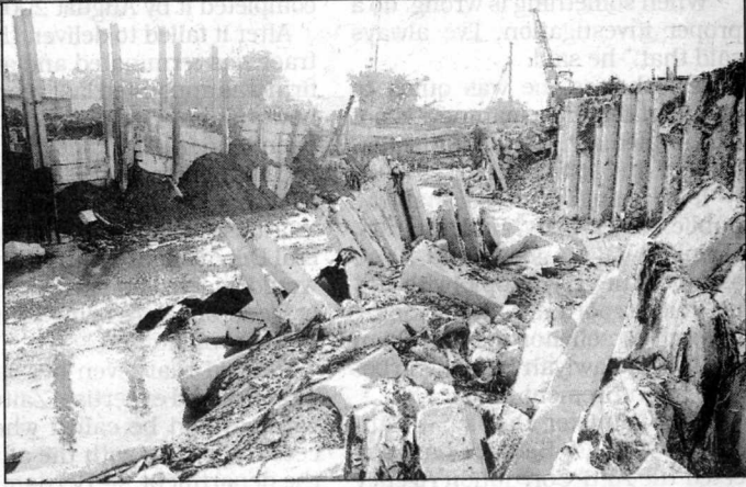
DUMPING GROUND: Indiscriminate dumping of debris along Sungai Kerayong is the primary cause of the flash flood
