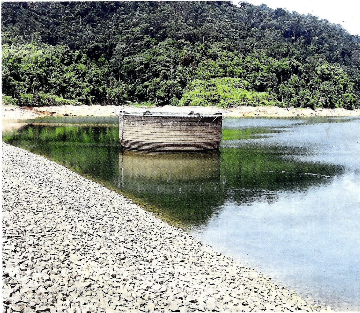
Bad sign: The water level at the Air Itam Dam in Penang reading 52.3% at 12.25pm yesterday.
