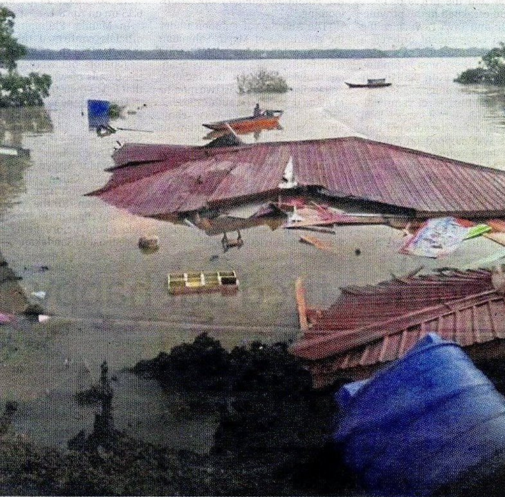
All that's left: Erosion at the riverbank caused parts of SK Kampung Buda in Spaoh to collapse and disappear into the Saribas River.
