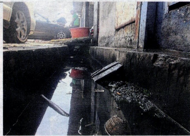
A drain clogged with oil grease and sludge found behind a shoplot.
