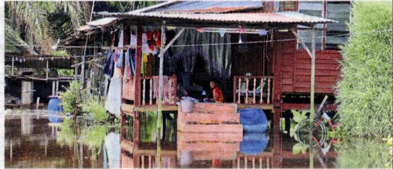
Water, water, everywhere: One of the houses that was affected by the floods around the Mukim Sri Gading area, near Ayer Hitam.
