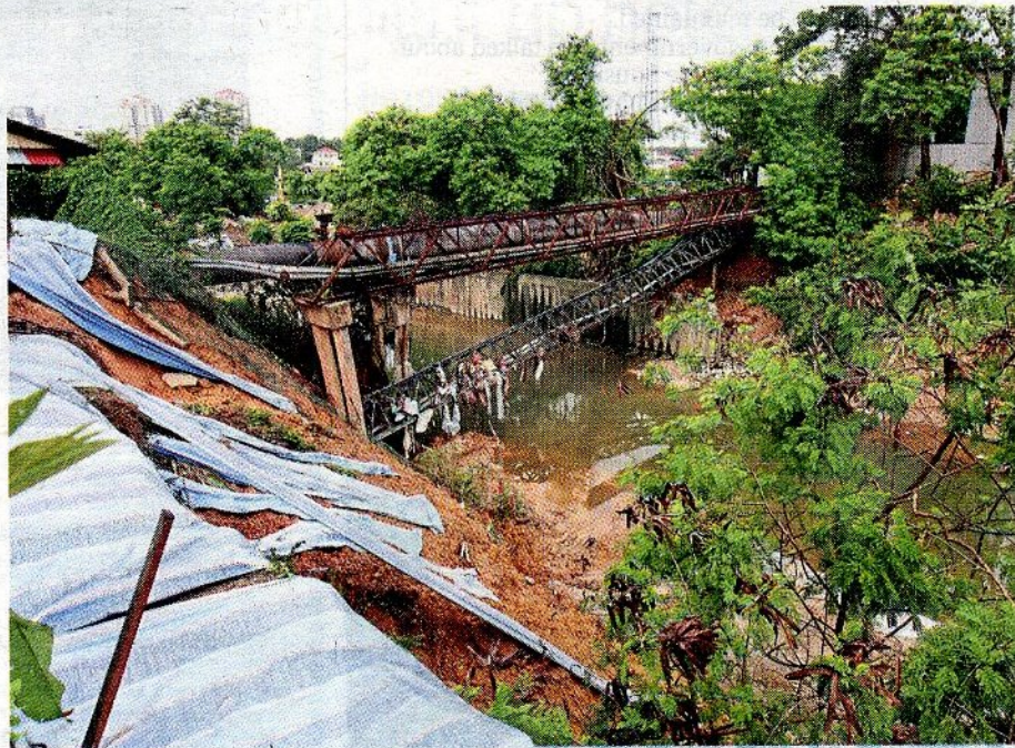
Work to repair the eroded riverbank is expected to start this week.
