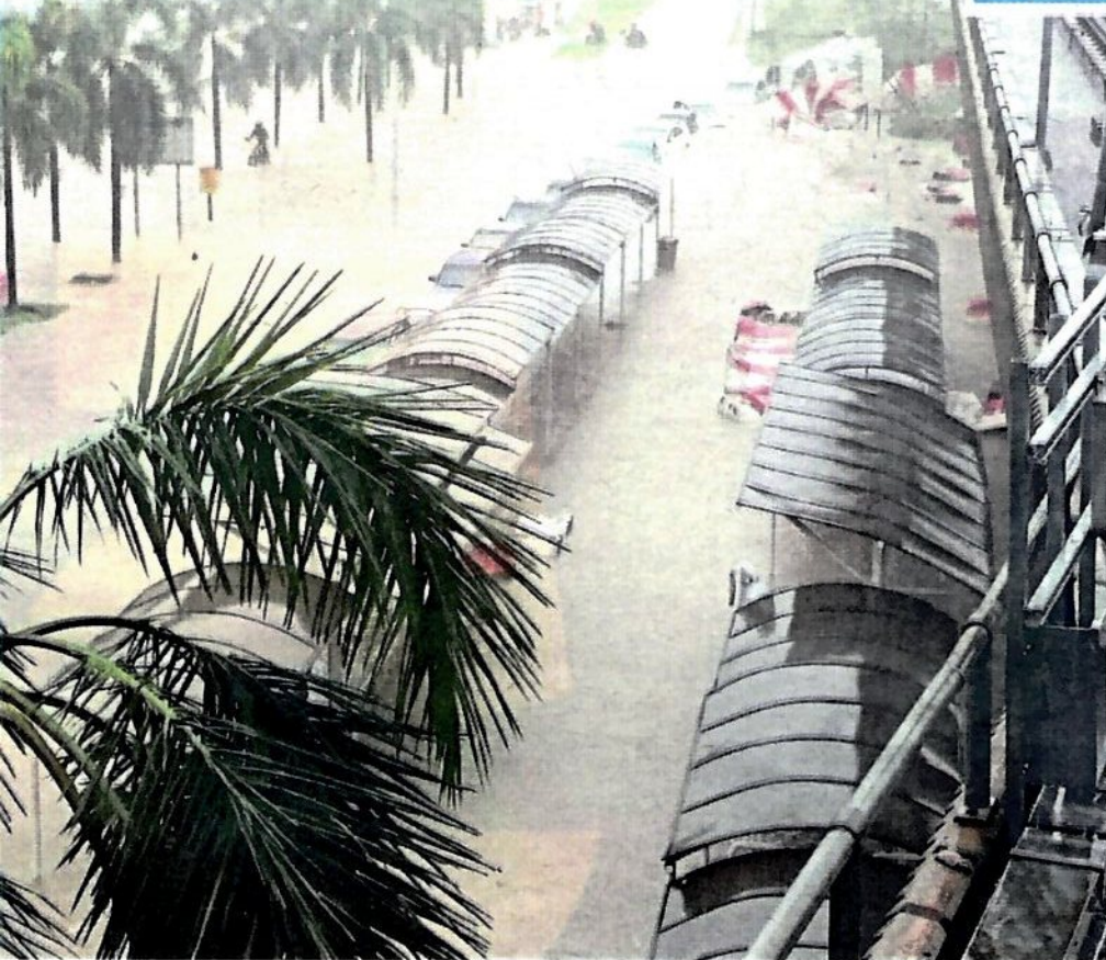
Flood woes: The Sungai Besi LRT station was inundated after a massive downpour.
