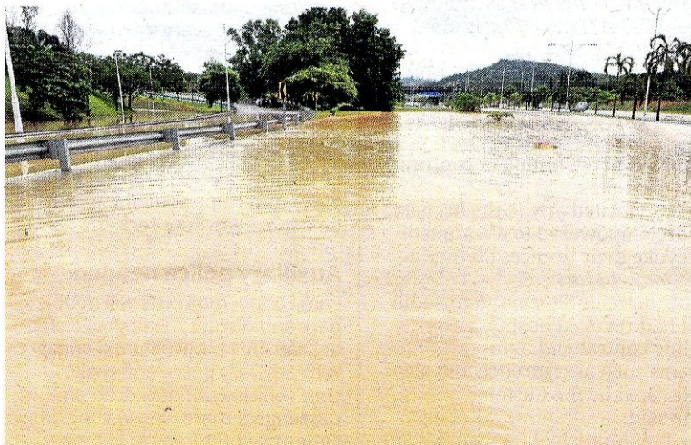
The downpour also affected roads in Putrajaya as Jalan Timur near Pinggiran Desa Putra from Putrajaya International Convention Centre towards Kuala Lumpur was flooded.
