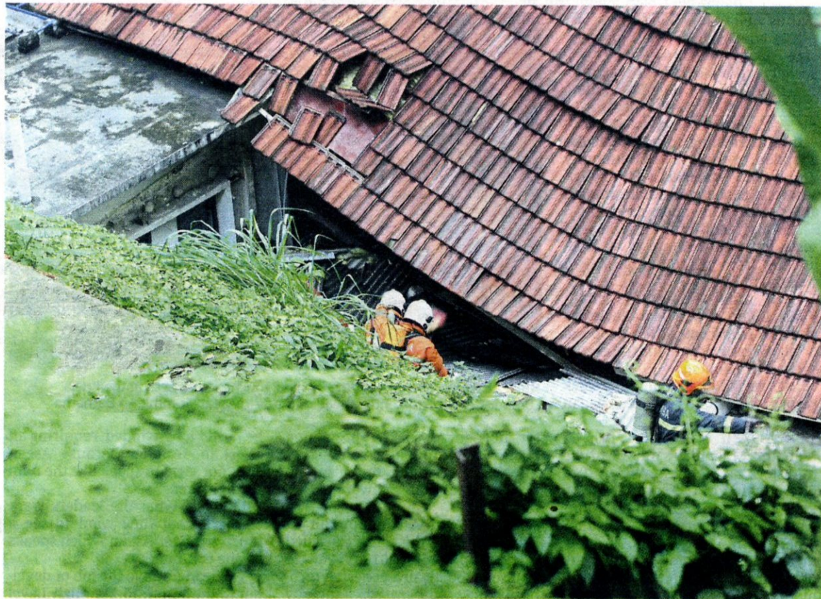
Safety checks: Kuala Lumpur Fire and Rescue Department personnel monitoring the area where a landslide caused damage to a restaurant in Jalan Raja Chulan. — Bernama
