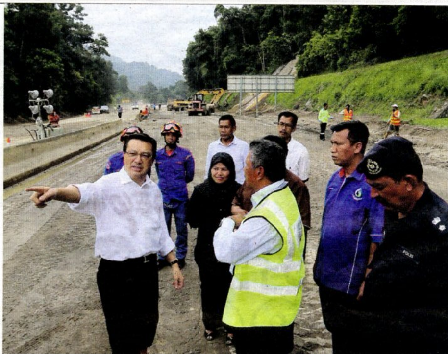
Transport Minister Datuk Seri Liow Tiong Lai surveying the site of the mudslide at Km52.4 of the Karak Highway yesterday. Pix by Abdullah Yusof and Ghazali Kori
