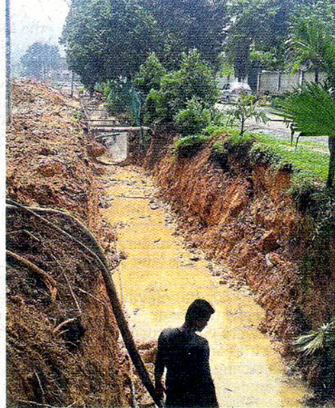
Workers constructing the U-shape concrete drains along a 200m stretch of the existing drainage in Pandan Glades, Ampang.
