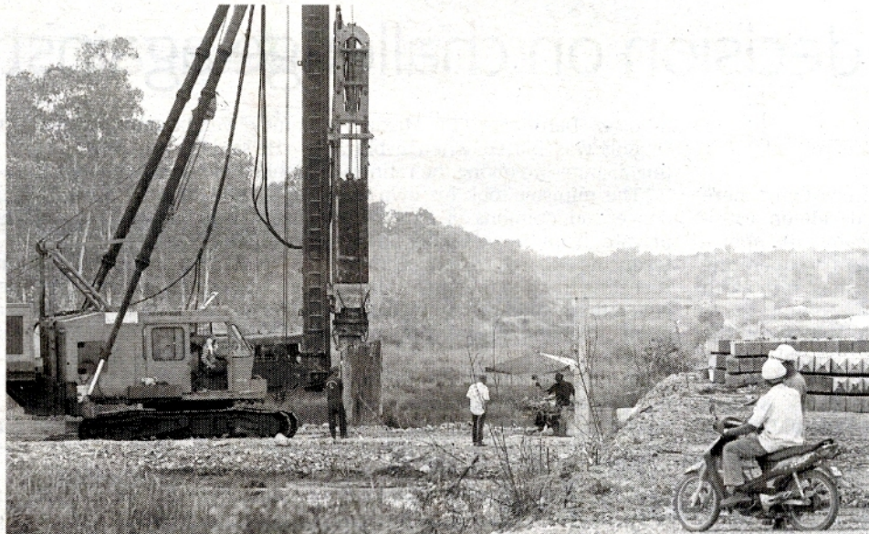
Work in progress: Work on Phase One of the Baroh Tok Jiring flood mitigation project going in Kuala Nerus.
