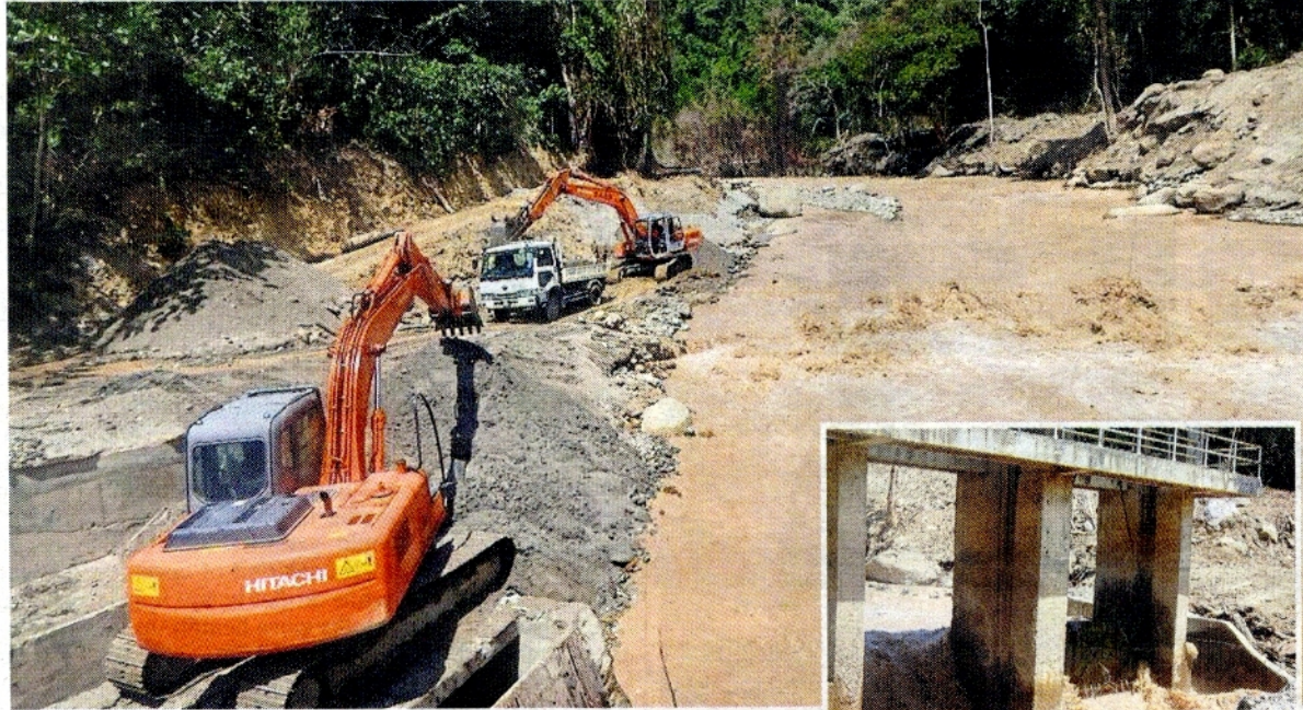
Ongoing effort: Officials trying to clear the silt after heavy mudflow into a water intake point in Ranau's Sungai Liwagu forced it to shut down (inset).
