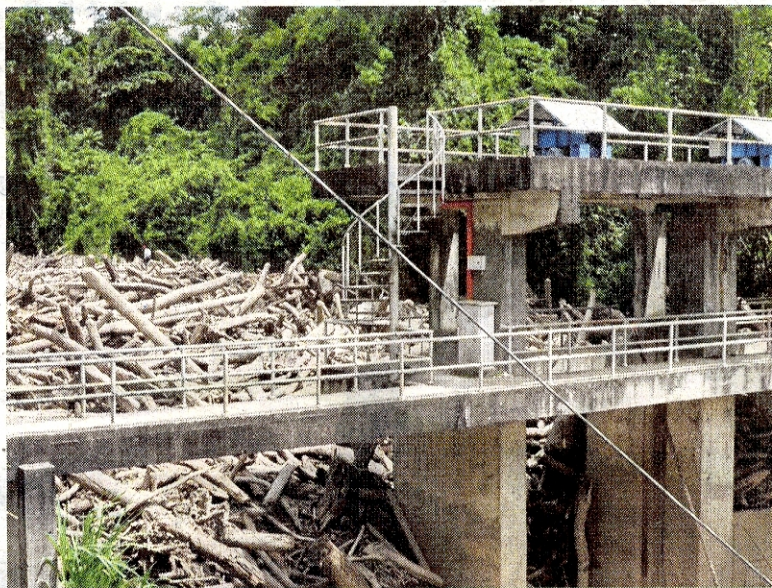
Clearing work at the Bambangan water treatment plant in Ranau started yesterday. Bernama pic
