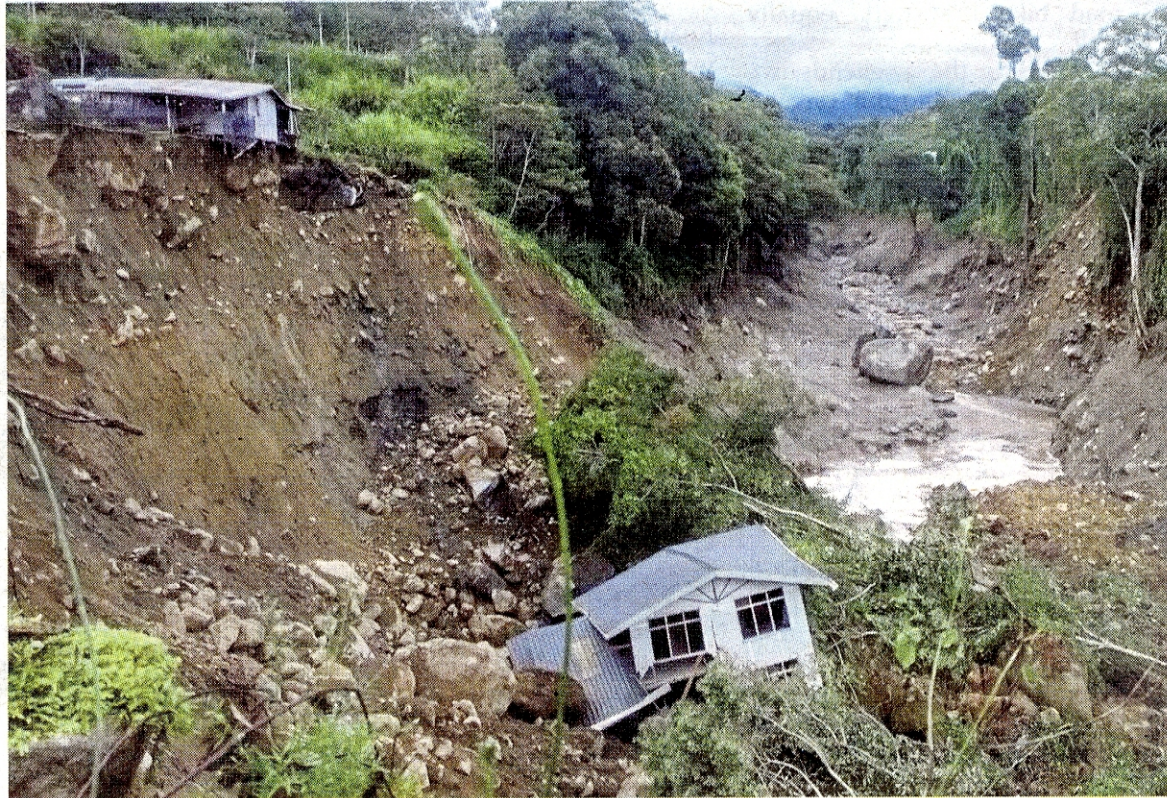
A house hanging precariously at a ravine in Kampung Mesilau, Ranau, yesterday. Pic courtesy of NST reader
