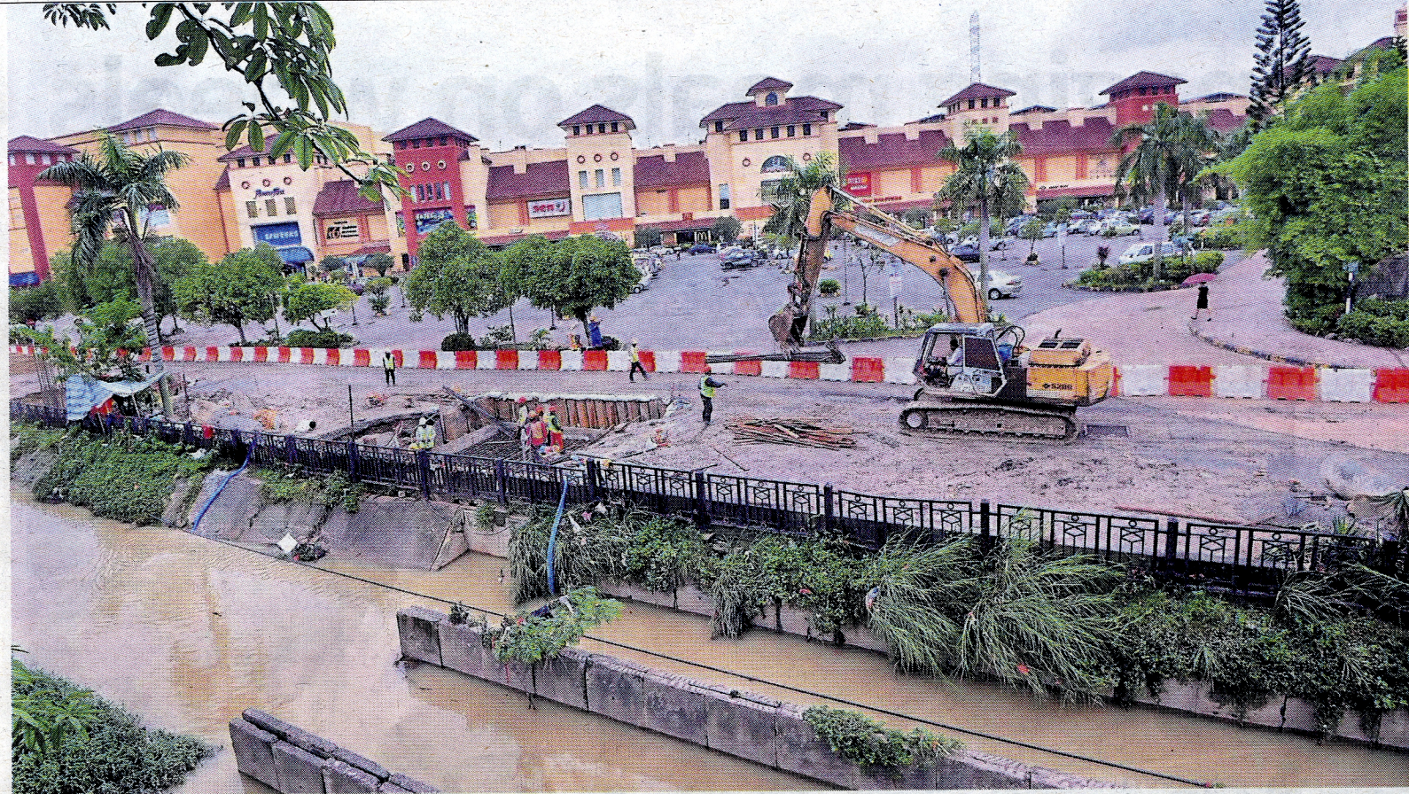
Clean-up: Workmen seen de-watering the LRT construction site in front of the flood-hit surface carpark at IOI Mall Puchong.
