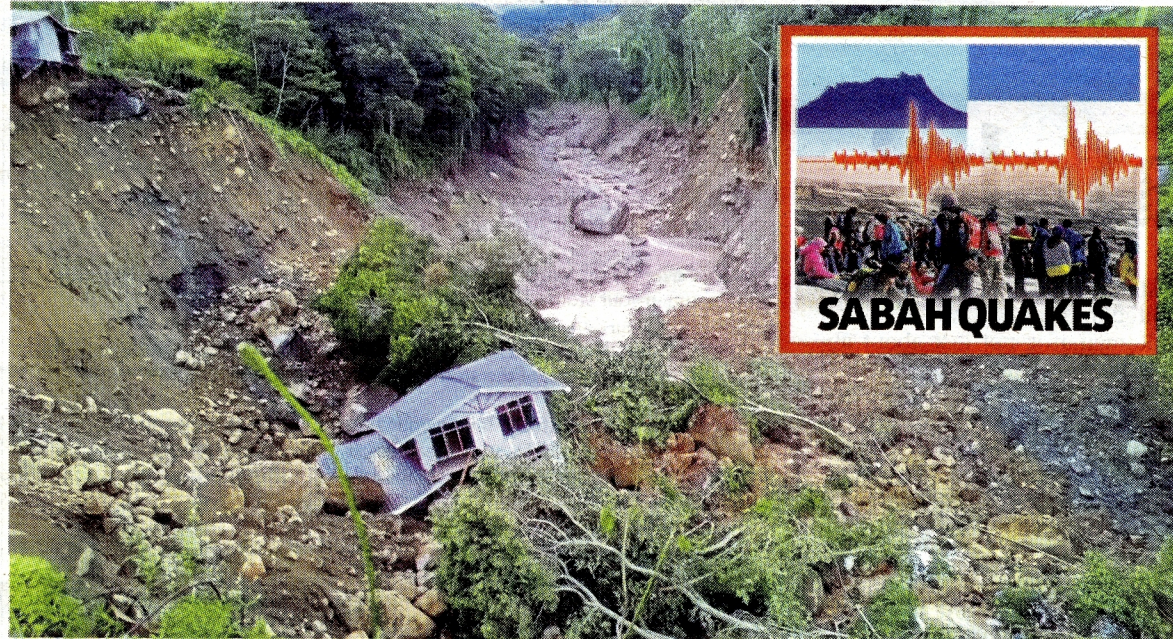
The nearly completed home of Jahili @ Haili Salim that came tumbling down due to mudslides near Sungai Mesilau in Kundasang, Ranau. Pic courtesy of reader
