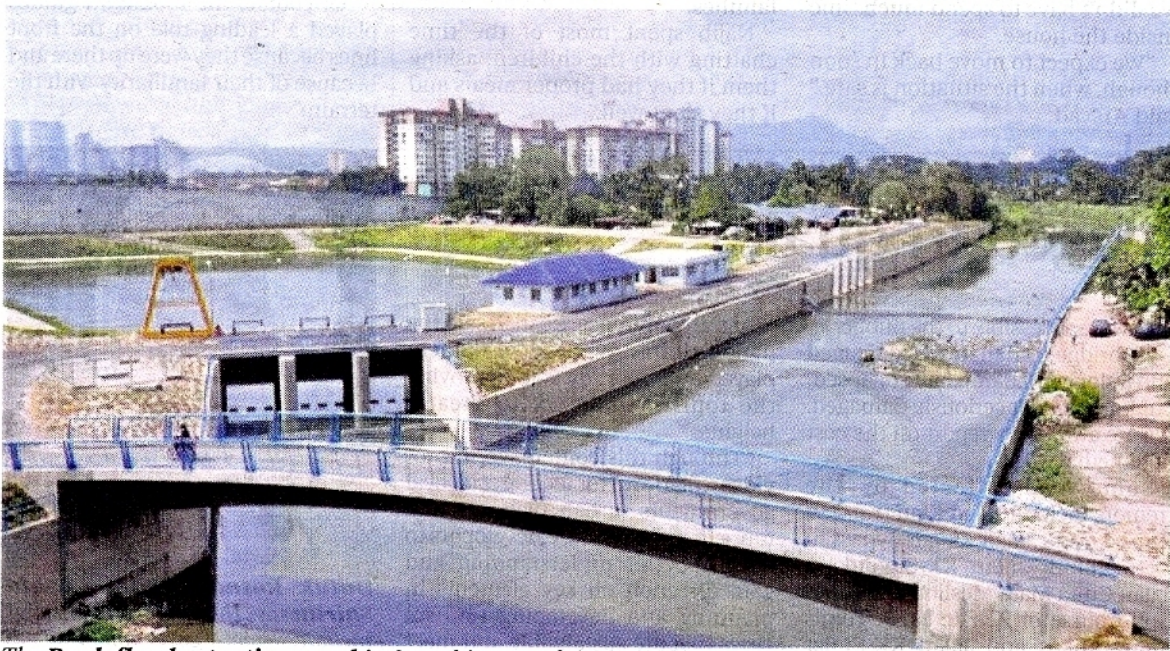
The Puah flood retention pond in Sentul is part of the 65 work packages in the River Cleaning phase .
