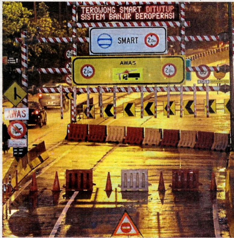
Temporary closure: The SMART tunnel being closed to traffic following a storm in Kuala Lumpur.
