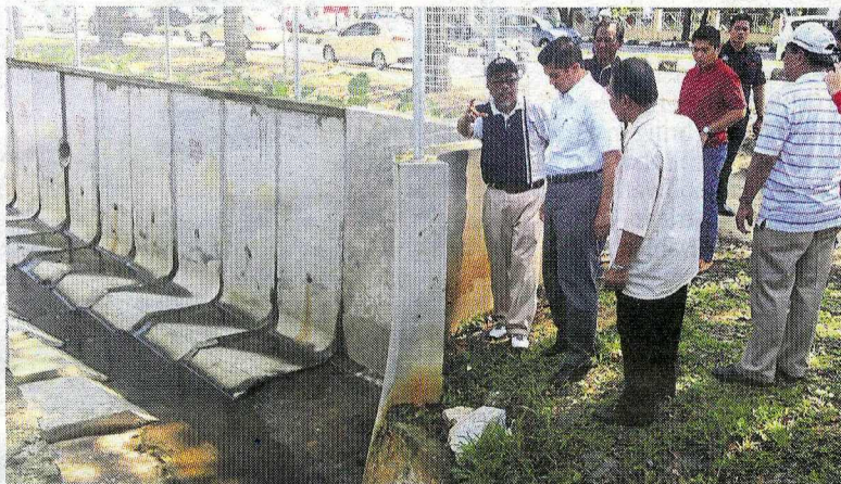
Site visit: Mohd Jaafar (left) briefing Azmin (second from left) on the various flood mitigation work being carried out by the council.
