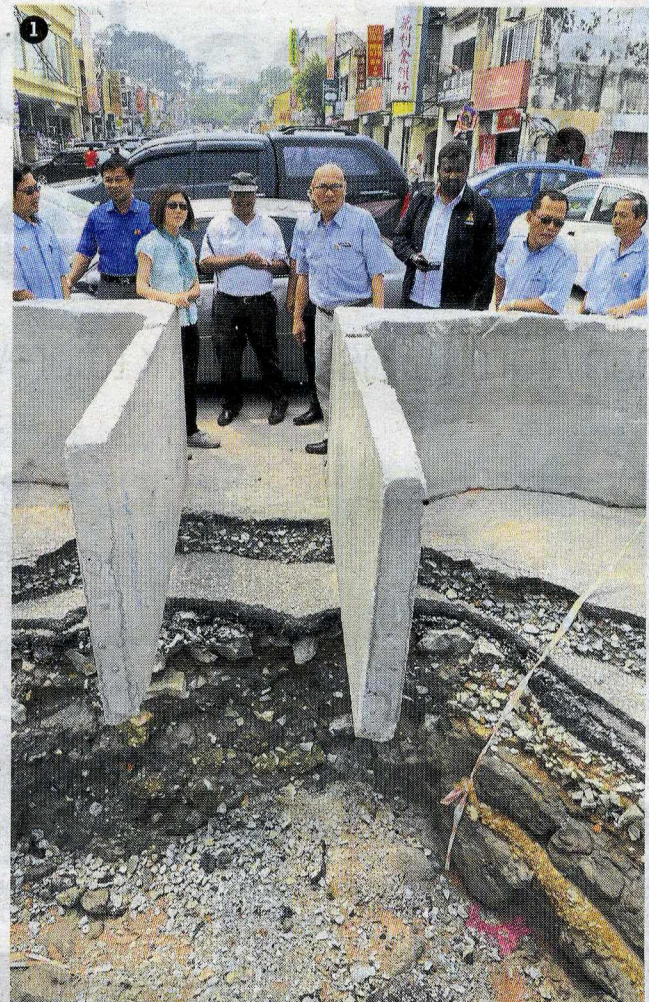
1 Gan (third from left) and Nor Hisham (fourth from right) inspecting a site for a drainage upgrading project, with JPS and MPS personnel in Rawang town.
