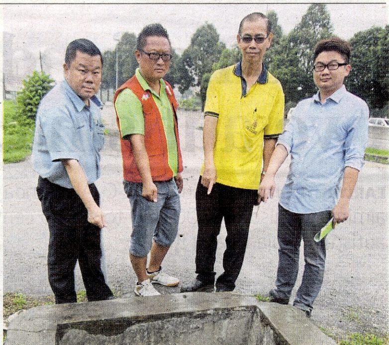
Loka Ng Sai Kai (left) and Serdang Lama residents point at the drain that will be widened and deepened . Pic by Mohd Khairi Ruslan
