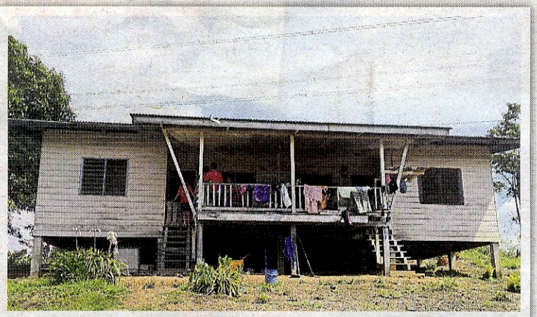
The volunteers lived in this house for ten weeks while building the GFWS. Before that, Kampung Lumou relied on rain as their primary source of water.
