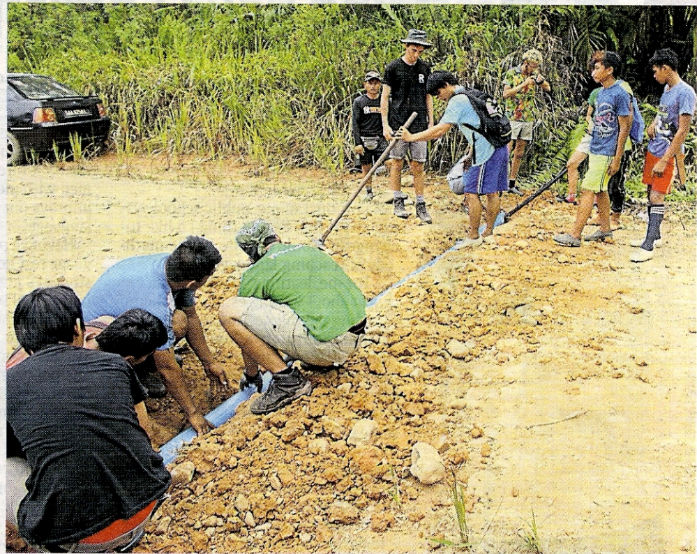
Volunteers laying the pipes that will bring water from the GFWS to the village.
