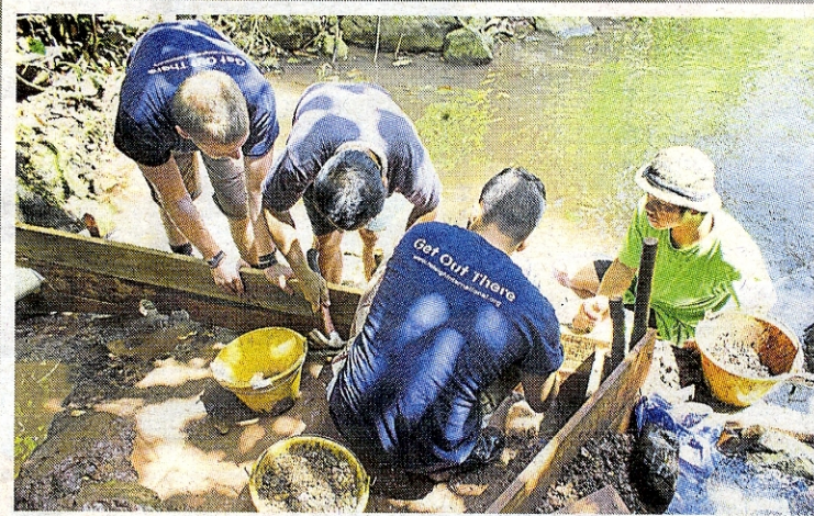
Raleigh International volunteers built a 'gravity-fed water system' (GFWS) for the people of Kampung Lumou. They are pictured here building a dam at the water catchment area which feeds the GFWS.
