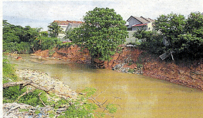
Choked river: Taman Cheras Jaya residents are worried that the river bank of Sungai Balak is eroding.
