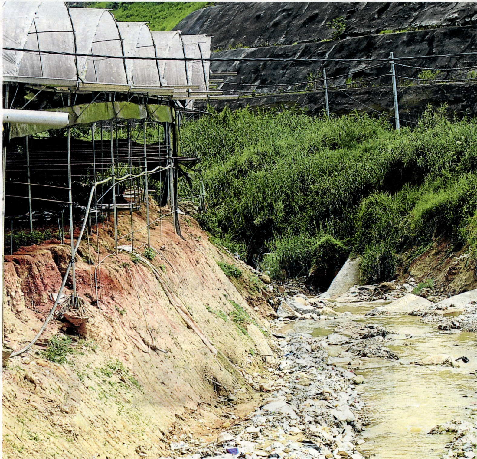
The Oct 23 flash floods that killed three people failed to serve as a reminder to the farmers in Bertam Valley. Almost every metre of the Sungai Bertam river reserve is dotted with rows of leafy greens and flowers. Pix by L. Manimaran
