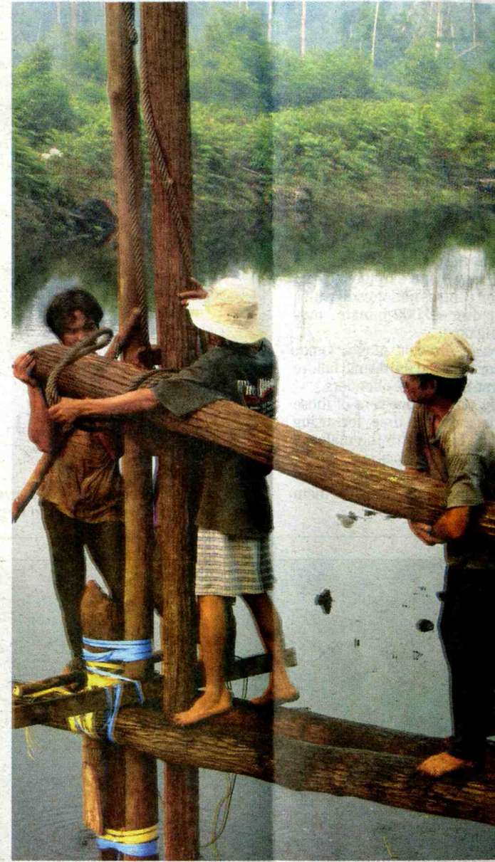
Local communities construct the blocks by hand in Central Kalimantan. — Picture by Yus Rusila Noor, Wetlands International.
