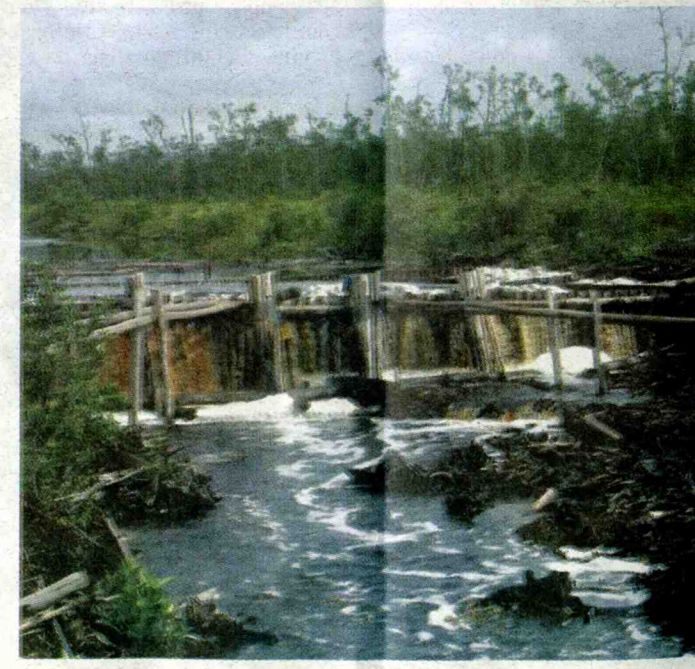
Local communities call these mammoth canals "hell canals" because they suck water from peatland, leaving them prone to horrible fires. This block in a Central Kalimantan canal keeps the water from flowing out. — Picture by Nyoman Suryadiputra.
