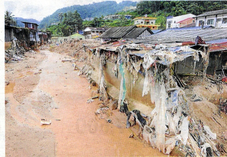
Risky riverside: The remains of homes washed away by the recent mud flood along the Bertam River in Cameron Highlands. — Bernama
