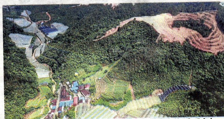
A swathe of bare land can be seen at the top of a hill in the Ulu Jelai area in Cameron Highlands.
