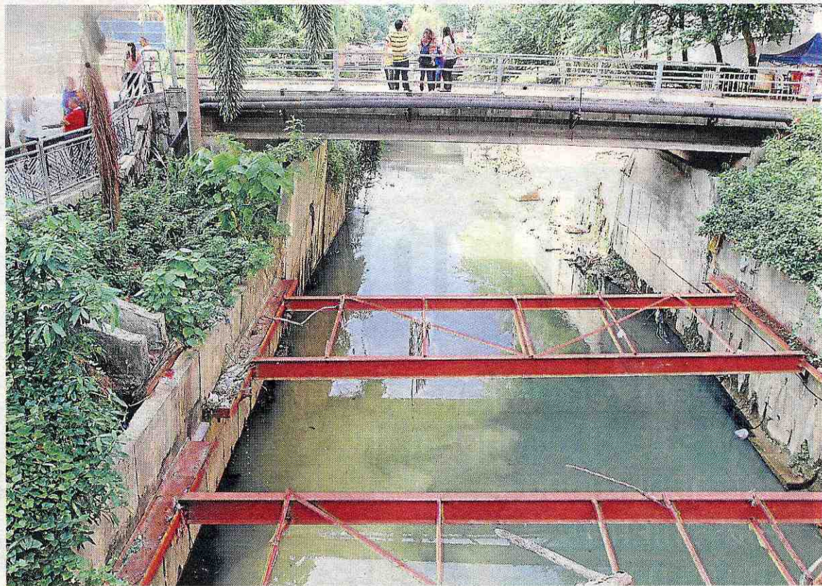
Remedial measures: MBPJ spent RM1mil to install steel sheet piles to strengthen the river walls after the road collapsed in 2011.
