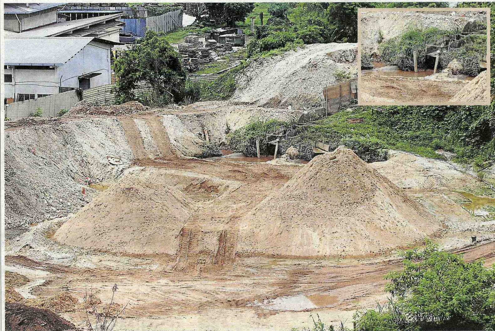
No activity: Although eyewitnesses claim that the site was in operation at 8am yesterday, the place was found to be abandoned when DBKL visited the site at 10 am. (Inset) The piping system that is connected to the Klang River.
