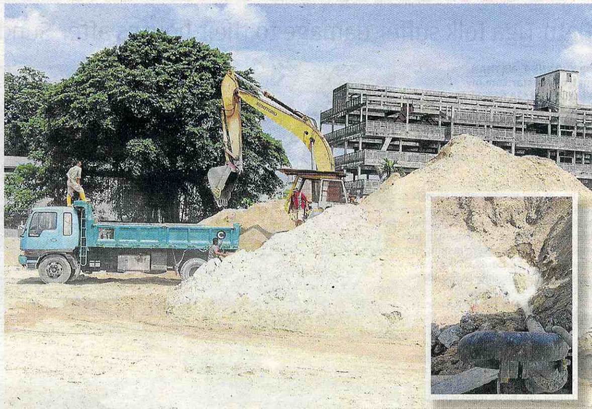
Routine: A lorry about to load washed sand. (Inset) Water being discharged back into the Klang River.
