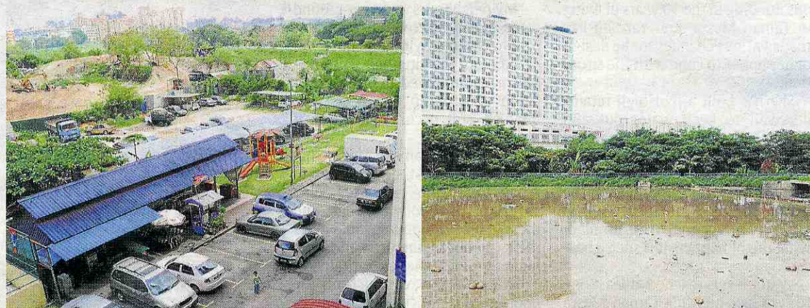
Too close for comfort: The close proximity of the sand-washing site (left) has been worrying the residents for years. (Right) An oxidation pond next to Seri Anggerik PPR which has not been working is also said to contribute to the stench and breeding ground for mosquitoes.
