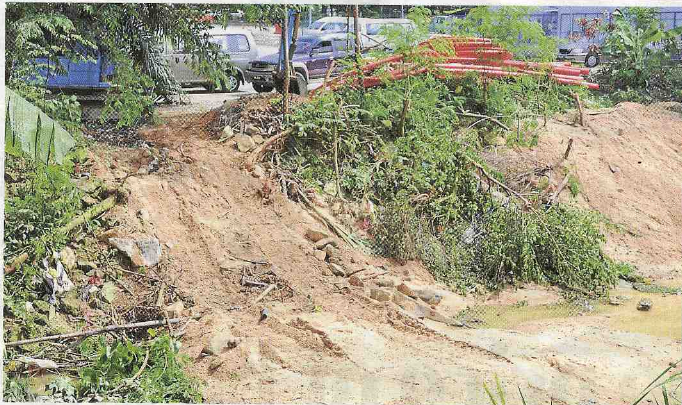
Wrong procedure Silt dredged from the bed is piled by the riverbank, raising concerns among residents that it will flow back into the river come next rainfall.
