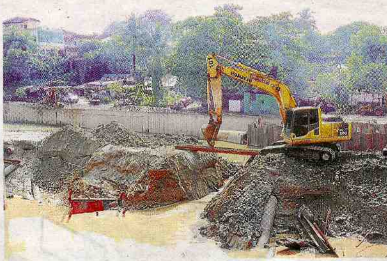
Work in progress: The River of Life project that is taking place along the riverbank of Sungai Gombak that cuts through Kampung Puah.
