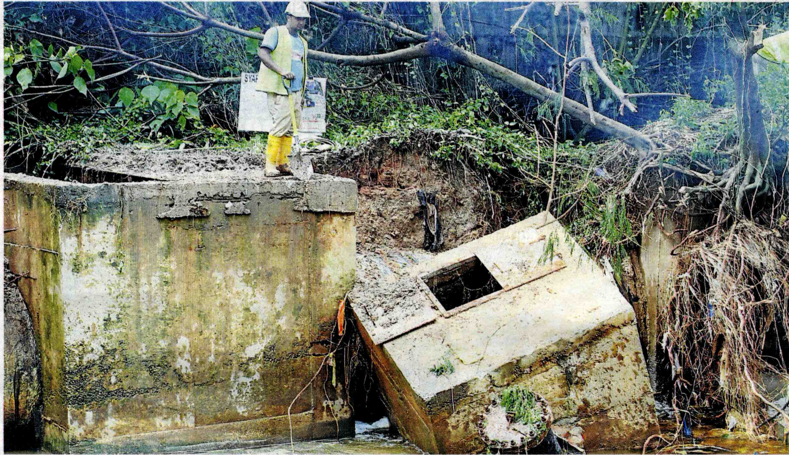
A Syabas worker at the Dusun Kubung pond at Batu Caves helping to remove a displaced water chamber and patch up the burst pipe. Pic by Mokhsin Abidin
