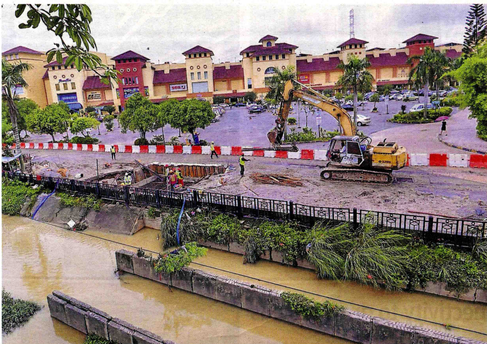
Clean-up: Workers de-watering the LRT construction site in front of the open-air carpark in IOI Mall Puchong yesterday morning, while some parts of the road remain muddy following the flash flood on Monday evening.
