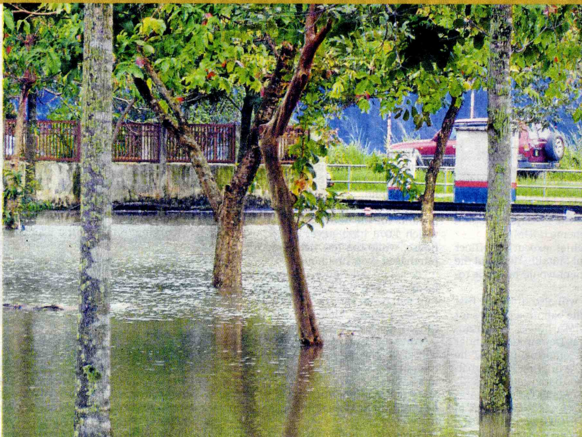
A proper drainage system is vital in flood-prone areas.
