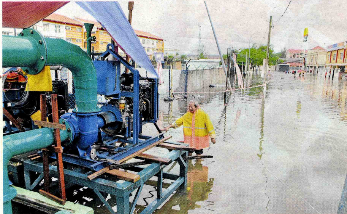
A Drainage and Irrigation Department worker checking on a water pump near Universiti Malaysia Kelantan in Kota Baru, Kelantan, yesterday. Some 2,000 students and staff of the university were affected by the flash floods that hit the area. Bernama pic
